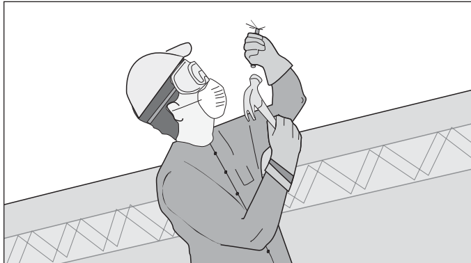
Fig.5. Make an initial hole.
