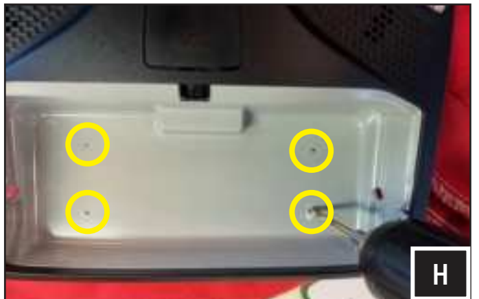
H. Use a 6mm drill bit to drill 4 holes.
