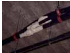
Support both sides of Y-joint and header.
