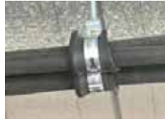
Additional piece of Insulation (prevent from insulation damage)
