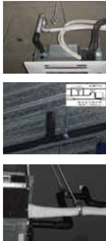
Sample of Good Installation
