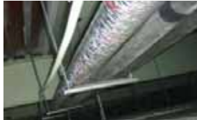
Saddle support or hanger can applied
