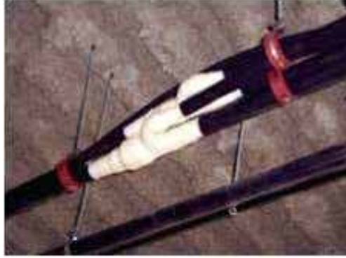
Support both sides of Y-joint & header.
